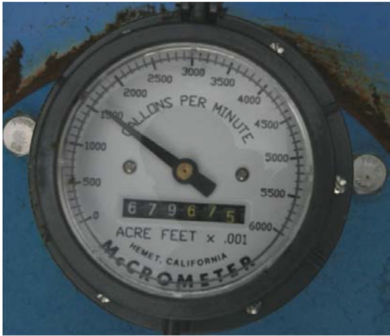
Figure 3: Example Flow Meter Display (Totalizer reads 679.675 acre-feet)
